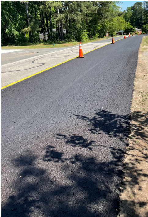
Pictured above: First course of Micro Surfacing on NC 109 in Wadesboro.
