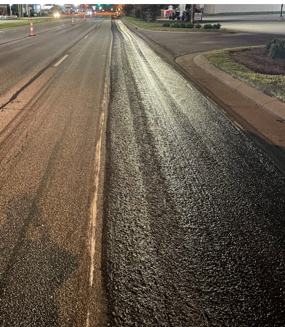
Pictured above: Rut fill course applied in right wheel path of US 74 WB in Monroe.
